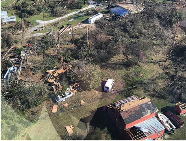
PHOTO COURTESY OF WEST FLORIDA ELECTRIC COOPERATIVE, FLORIDA
